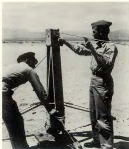
A hand winch is used to position the barrier.
