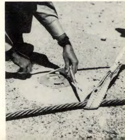
Anchor, lifter strap combine to lift cable.
